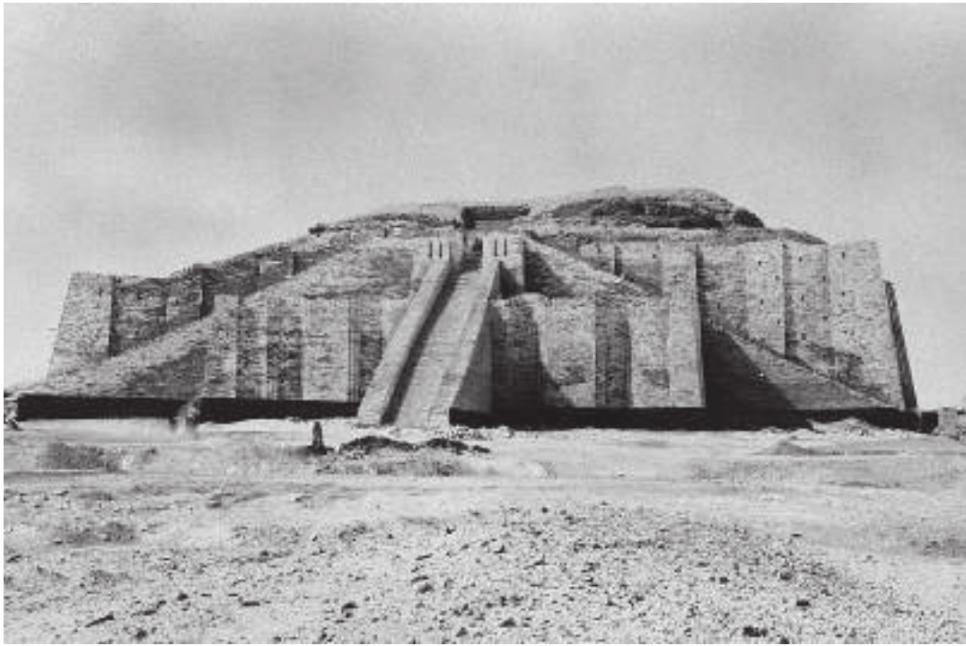
Northeastern facade (the ascents partly restored) of the ziggurat at Ur, southern Iraq. Hirmer Fotoarchiv, Munich
