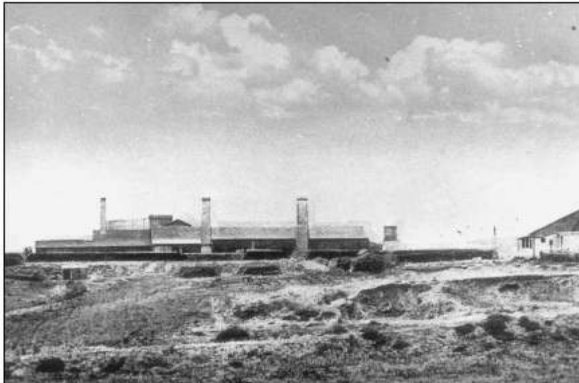
LA BOLSA TILE COMPANY LOCATED AT GOTHARD AND ELLIS, C. 1910. At one time, this became the largest clay tile factory west of Chicago, and provided year-round employment for many Huntington Beach residents.
