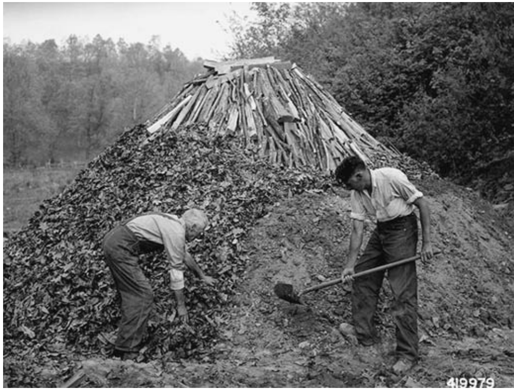
Figure 3.3 Preparing for charcoaling, June 1942, Wayne National Forest, Ohio. C. A. Masie (left) and David Daniels putting wet leaves and then dirt over the wood to restrict oxygen so that burning will produce charcoal. An immense amount of wood was used to make charcoal.
