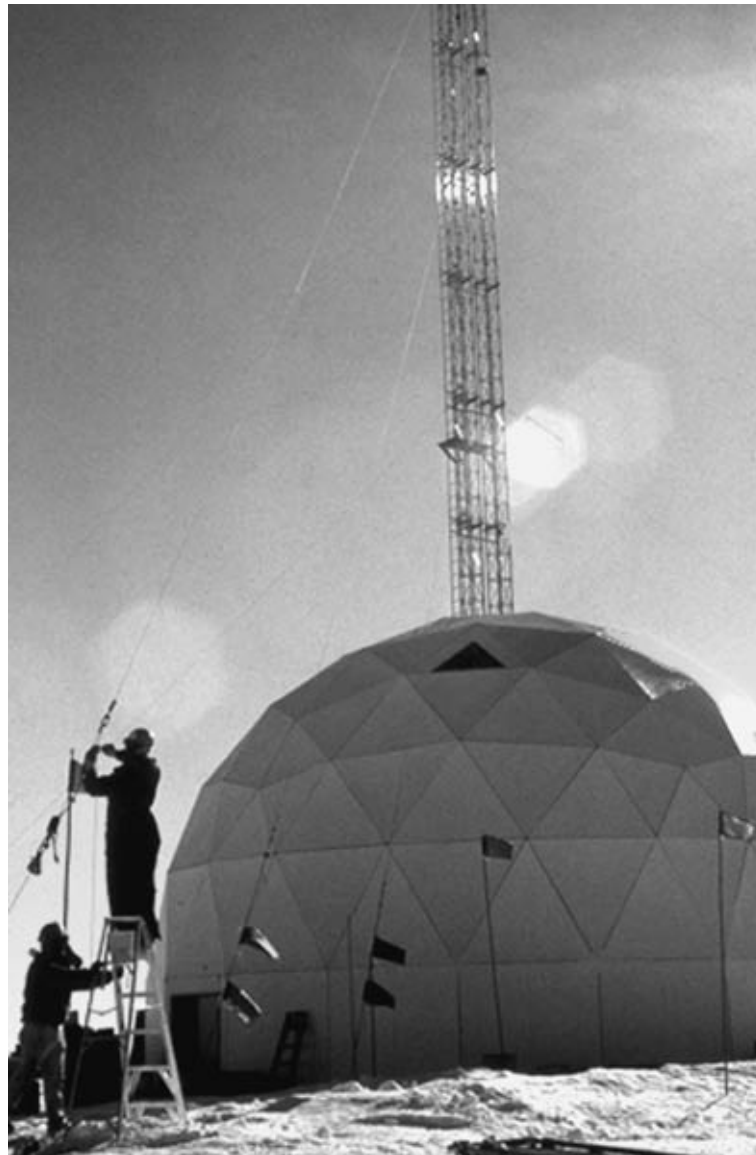
Figure 1.2 Final assembly of the drill and protective dome for deep ice coring at GISP2 in central Greenland. Records from ice cores tell us the history of the atmosphere, including natural and human-caused changes.
