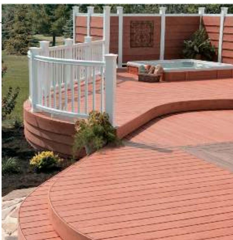
Deck builders make use of modern technology in the form of hidden deck fasteners and low- or no-maintenance synthetic decking. This deck uses both, with curving fascia boards that attractively conceal the structural components of the deck, and a built-in privacy screen around the spa tub that will never need to be painted or refinished. This deck will look just as new years from now, and requires very little maintenance on the part of the homeowner.
