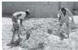
Fig. 2: Earth Mixing with cob and sand
