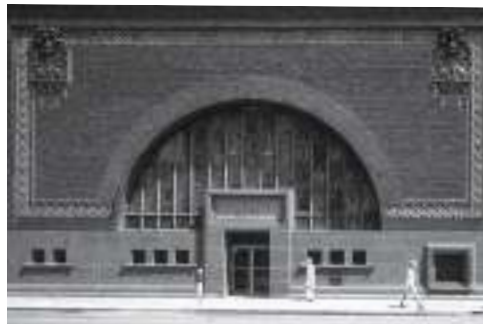
Fig. 6: Decorated brickwork Louis Henry Sullivan: National Farmers' Bank, Owatonna (USA), 1908
