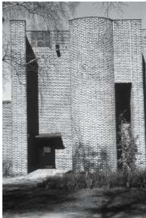
Fig. 10: Bed joint widths approaching the height of an individual brick Sigurd Lewerentz: Markus Church, Björkhagen near Stockholm (S), 1960
