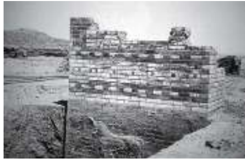
Fig. 2: The wall as a boundary element is the primary function, the masonry as loadbearing element the secondary function. Nineveh, excavations of town walls between 1899 and 1917
