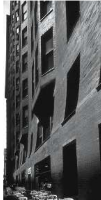
Fig. 11: The world's tallest self-supporting brick facade Burnham & Root: Monadnock Building, Chicago (USA), 1884–91, expanded by Graham, Greenwald and Roche, 1893
