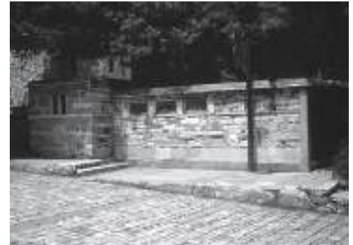
Fig. 8: The interweaving of the structure and its surroundings Dimitris Pikionis: Landscaping and refurbishment of St Dimitris Lumbardiaris Church, Philopappos hill, Athens (GR), 1957
