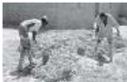
Fig. 2: Earth Mixing with cob and sand
