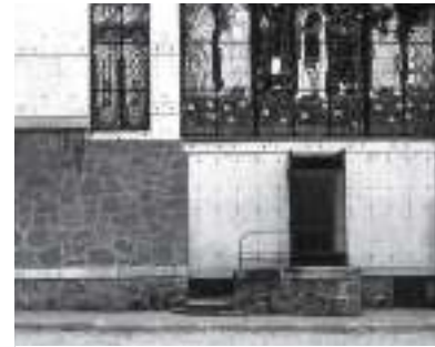
Fig. 4: Stereotomy and marble-clad masonry Otto Wagner: Steinhof Church, Vienna (A), 1907
