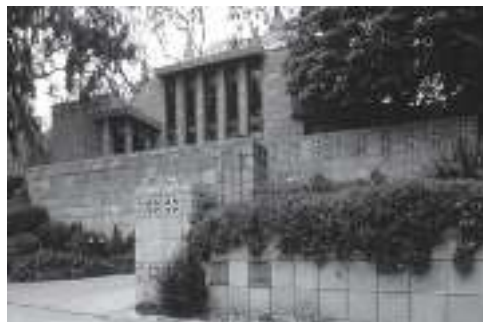
Fig. 7: Wright's second "textile block" house in Los Angeles Frank Lloyd Wright: Storer Residence, Hollywood (USA), 1923
