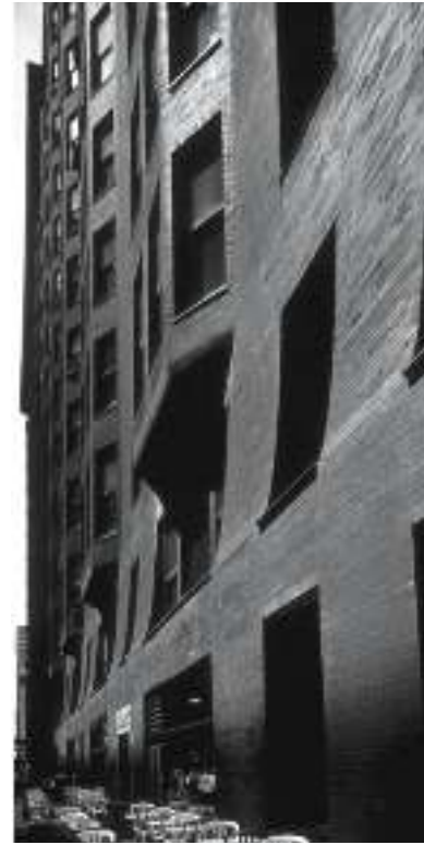
Fig. 11: The world's tallest self-supporting brick facade Burnham & Root: Monadnock Building, Chicago (USA), 1884–91, expanded by Graham, Greenwald and Roche, 1893
