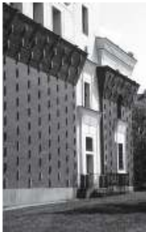
Fig. 3: Lightweight rendered facade over heavyweight masonry Jozef Plečnik: Sacred Heart of Jesus Church, Prague (CZ), 1939
