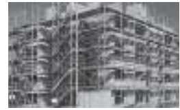
Fig. 5: Structural shell Masonry building, under construction
