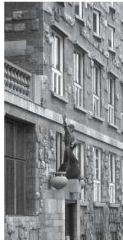
Fig. 5: A weave of natural stone and clay bricks Jože Plečnik: University Library, Ljubljana (SLO), 1941
