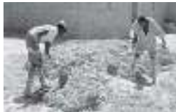
Fig. 2: Earth Mixing with cob and sand
