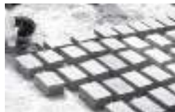
Fig. 3: Clay bricks Production, natural drying (in the air), Pakistan
