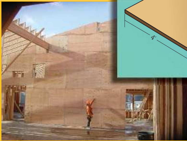
The engineered panel products on this wall provide the strength needed for the high ceiling of this elementary school.
